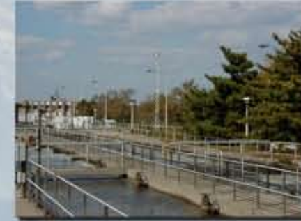
New York City Department of Environmental Protection Vertical dispersion curves were developed based on the controlled release of dual tracer gases for 77 separate process-tank monitoring events to support development of a refined hydrogen sulfide emissions inventory at a large NYC municipal wastewater treatment plant. Performed to address regulatory requirements in connection with a $500+ million facility upgrade, this work facilitated the site-specific customization of AERMOD – USEPA's latest guideline air dispersion model.
