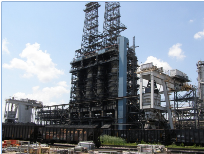
Figure 1. Houston Refining 737 Coker Unit
