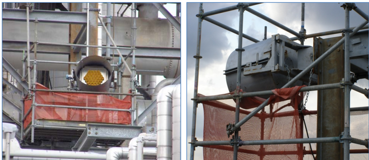
Figure 6. Retro-reflector Mirror Assembly, Front and Rear Views
